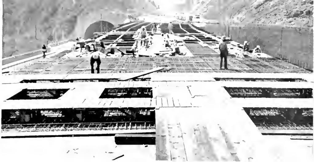
Steel construction on bridge section fast approaching completion
